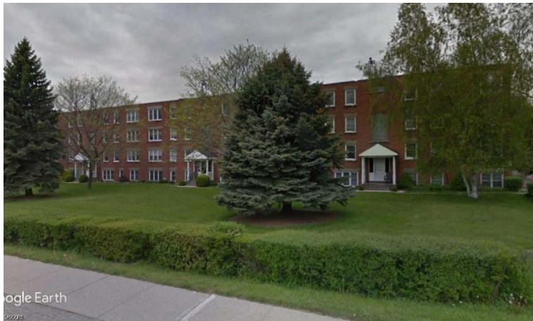
Figure 2b: Looking northwest at existing site
