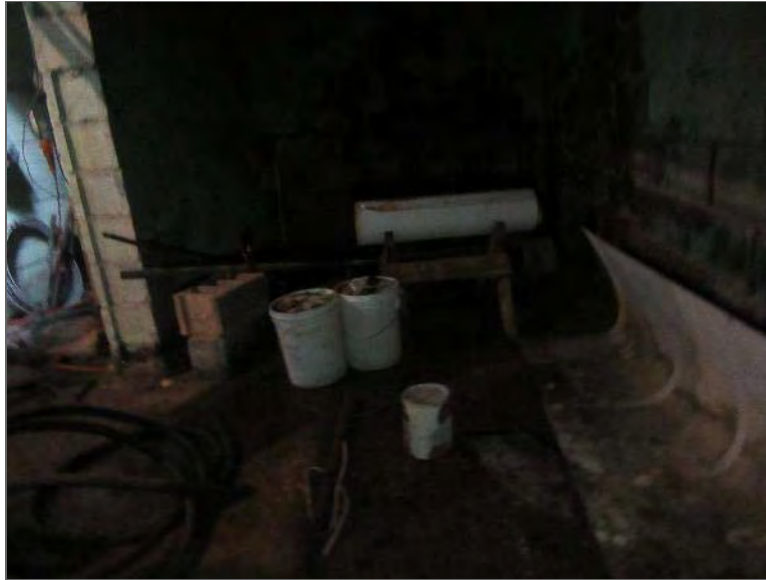
Photo 8 – Former coal storage area, located in the basement located within Site Building C.
