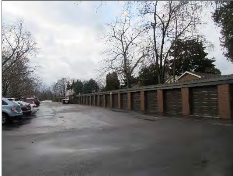
Photo 5 – General exterior view of Site Building C (east elevation looking west).
