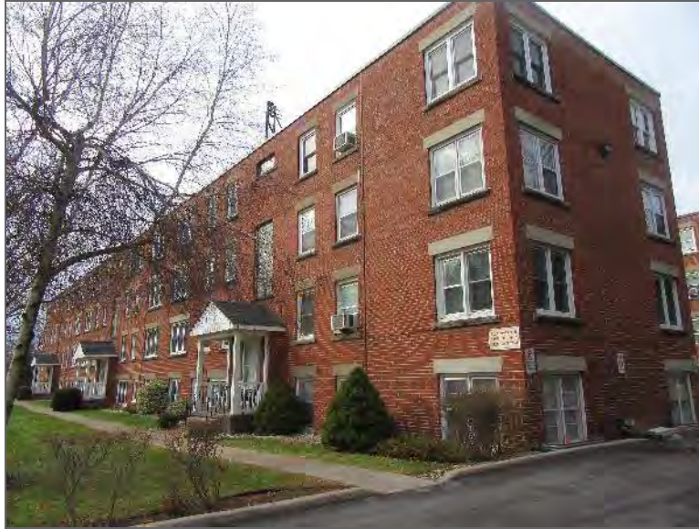
Photo 1 – Northwest and northeast elevations of Site Building A, looking northwest.
