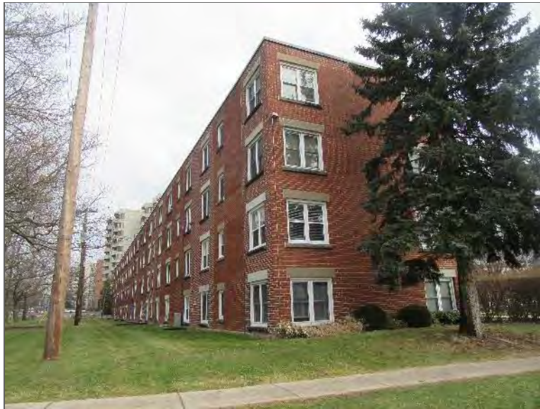
Photo 4 – Northwest and southwest elevations of Site Building B, looking northeast.
