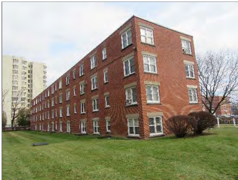
Photo 2 – Northwest and southwest elevations of Site Building A, looking southeast.
