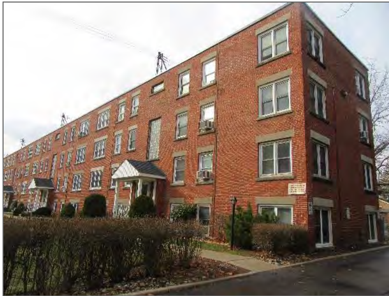
Photo 3 – Northeast and southeast elevations of Site Building B, looking northwest.
