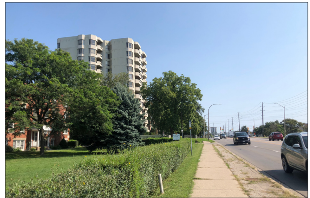
Subject site, view looking east from North Shore Boulevard
