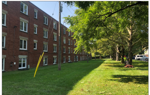
Subject site, rear view
