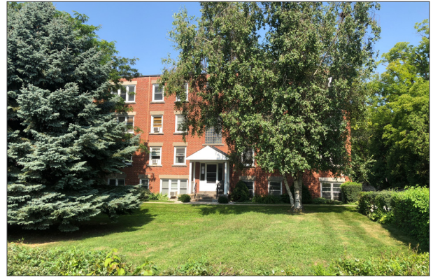
Subject site, view from North Shore Boulevard East
